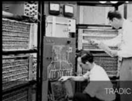
1956 TRADIC 700 transistors, 10 000 diodes
